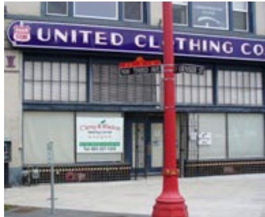
Our present location at 3rd and W Burnside in the historic United Clothing Building
